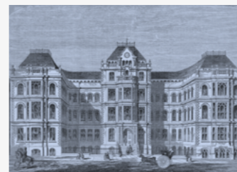
Adams Lace Warehouse, Stoney Street, built 1855 and designed by T. C. Hine (courtesy of Nottingham City Council & www.picturethepast.co.uk)
