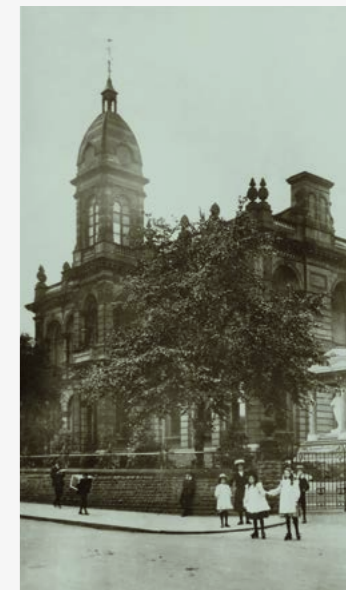
College of Art & Design, Waverley Street, built 1863-5 and designed by Frederick Bakewell of Nottingham (courtesy of L. Cripwell & www.picturethepast.co.uk)
