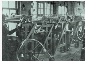
How the industry started: machines driven by hand similar to the early hosiery trade (courtesy of Nottingham City Council & www.picturethepast.co.uk)
