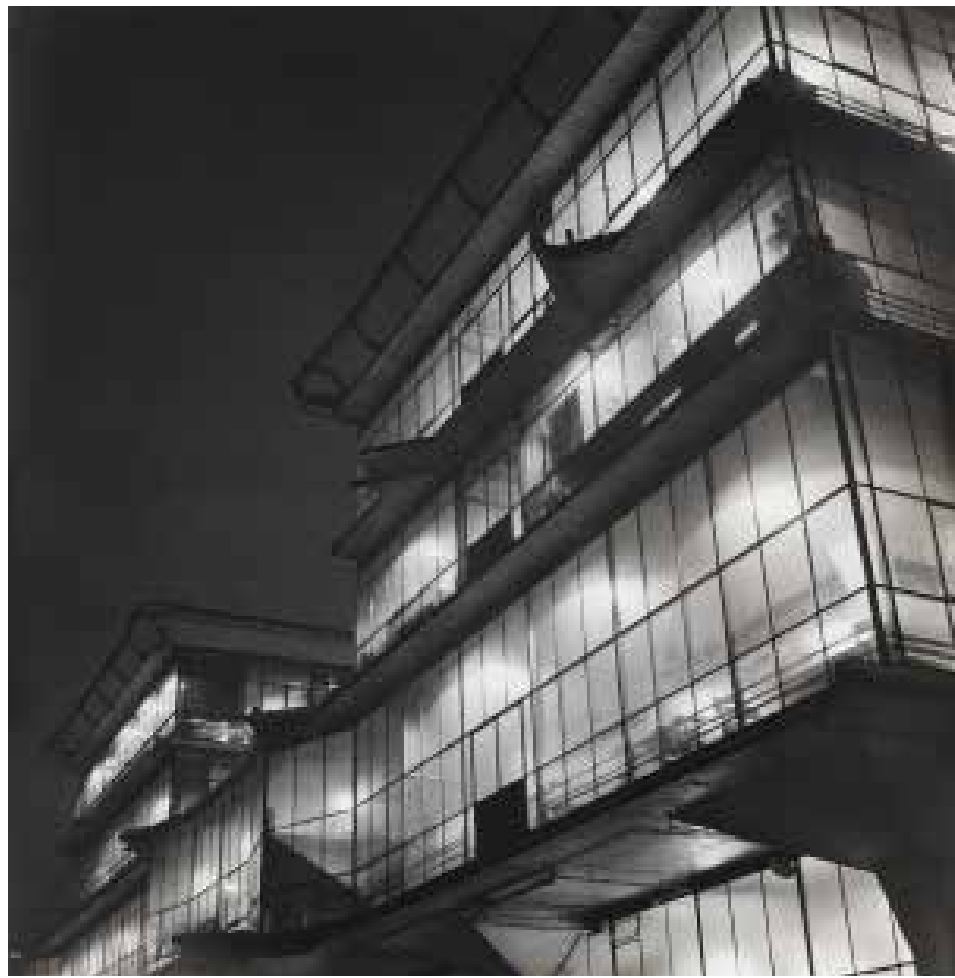
Left: the north side of the Boots D10 factory, near the dispatch loading bay. The jagged spurs were designed to connect to a possible extension, while the projecting rails supported window-cleaning equipment. Right: Women packing boxes on to the overhead conveyor in D10 (c.1935) – notice the male overseer. The horizontal conveyor system was removed prior to listing in 1971
