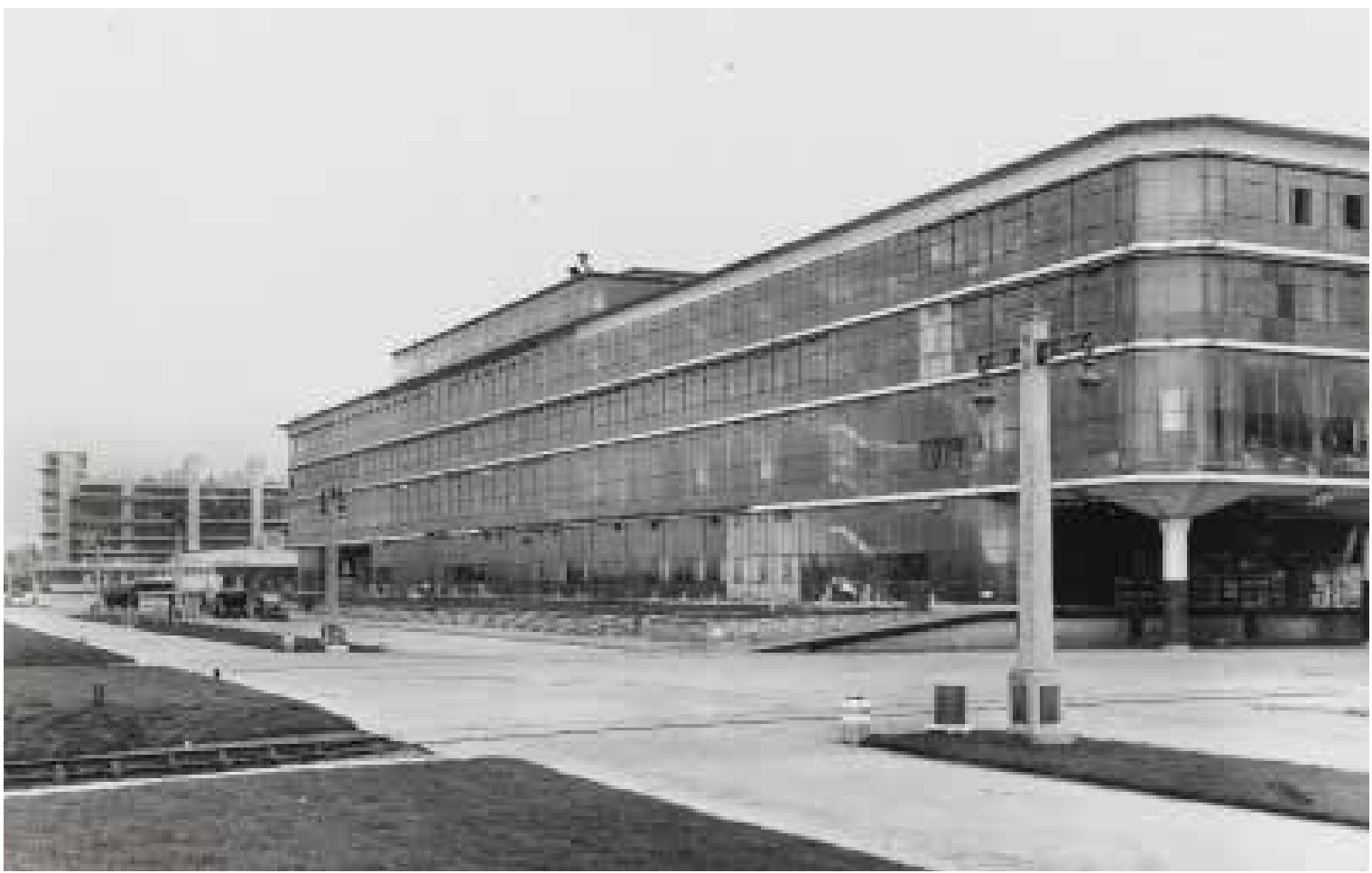
Left: Delivery dock south of D10, showing cantilevered shelter with travelling crane beside railway and wagons. Trains ran either side of the building as well as through it via a tunnel. The railway and steam engine were removed prior to listing.
