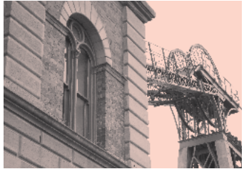
The restored winding engine house
