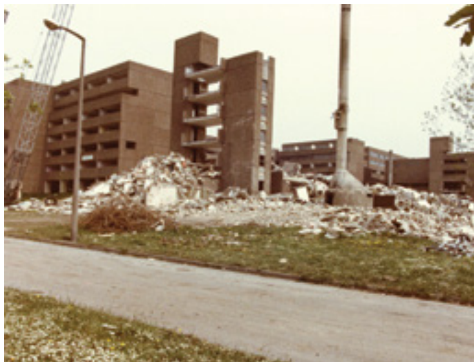
↓ Balloon Woods demolition under way, 1984 (Courtesy Reg Baker and www.picturenottingham.co.uk )
