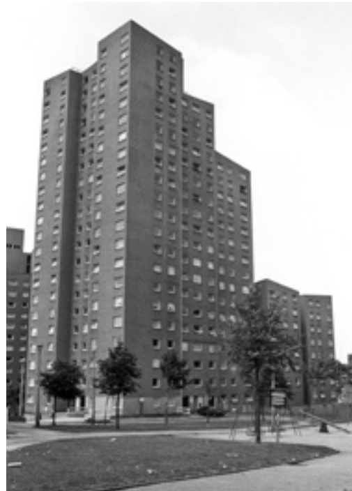
← Wimpey-built flats in Radford, previously nicknamed the '4B's', officially Buckland Court, Bladon Court, Bampton Court and Broadway Court. Renamed 'The Woodlands' following Estate Action refurbishment in the 1990s (Courtesy Reg Baker and www.picturenottingham.co.uk )
