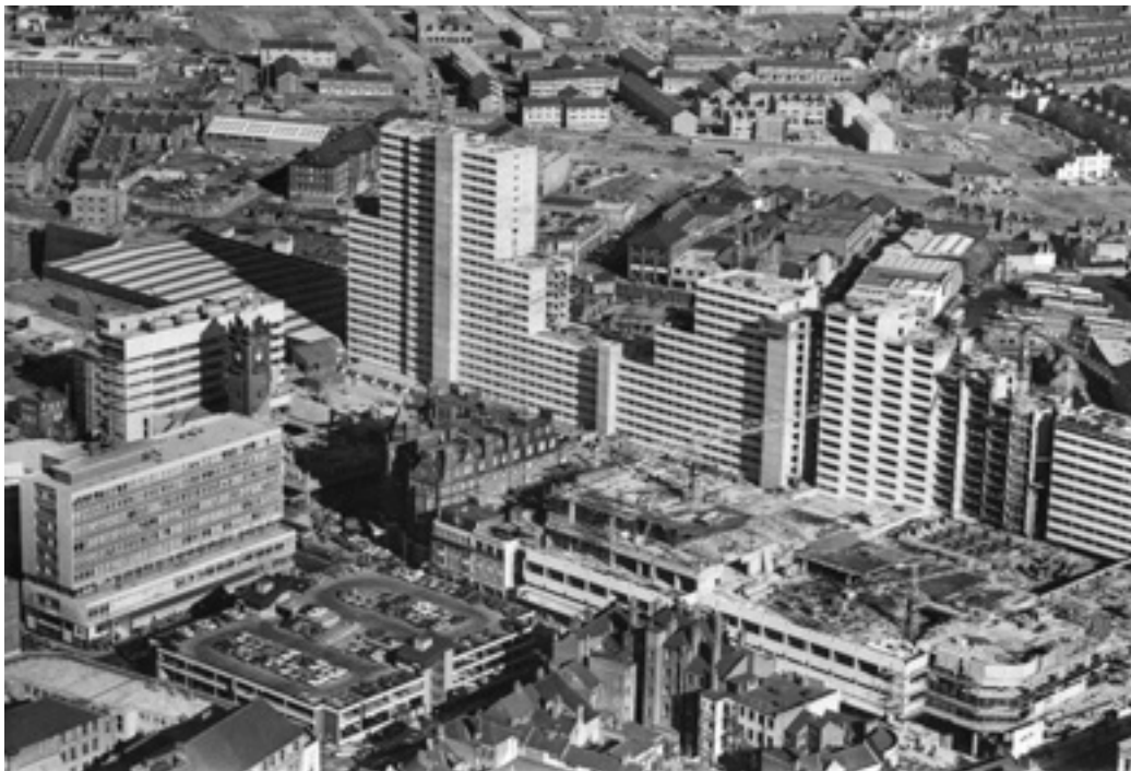
← The Victoria Centre Flats nearing completion (Courtesy Nottingham Evening Post and www.picturenottingham.co.uk )
