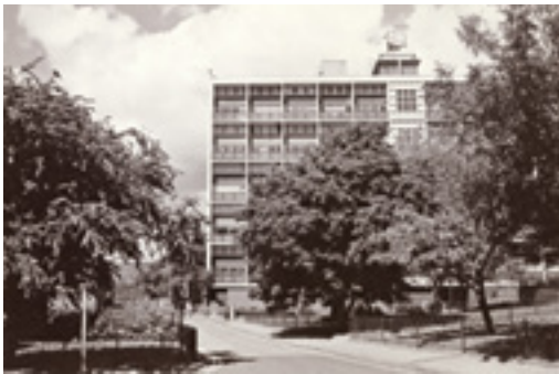
← Highcross Court, Radford, 1963: a concrete wall-framed block containing 112 maisonettes and built on a clearance site (Courtesy Nottingham City Council and www.picturenottingham.co.uk )
