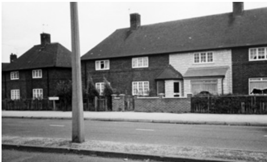
↑ An early Right to Buy house: notice a new brick wall, window, door and the faux stonework (Courtesy Nottingham City Council and www.picturenottingham.co.uk )
