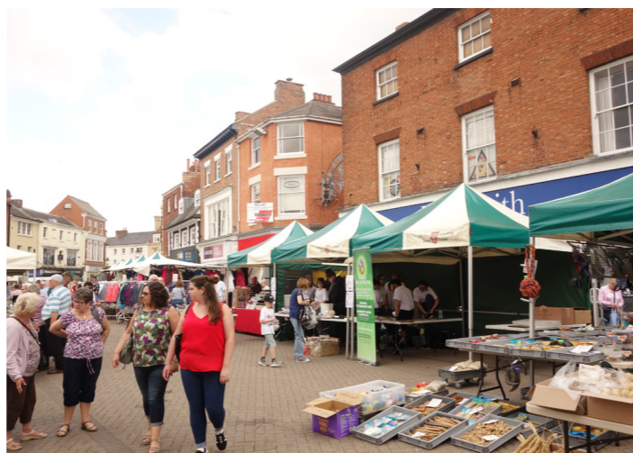
↖ The Market Place looking towards the South Parade/High Street entrance. In the foreground are numbers 29/29a. Notice the Georgian Sash windows with flat arched brick lintels above.
