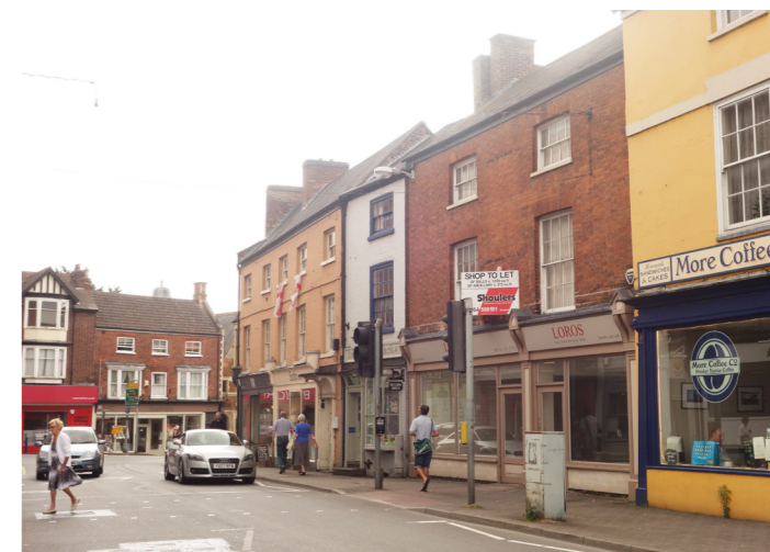
↑ The southern side of Market Place, showing numbers 10-16. Built at varying stages during the Georgian period with later Victorian and Edwardian shopfronts. Notice the reinstated shopfront of Loros.
